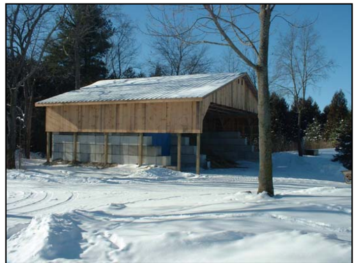
Manure Storage Project, Hop Hill Stable, Uxbridge. Photo by Nadine Abrams.
